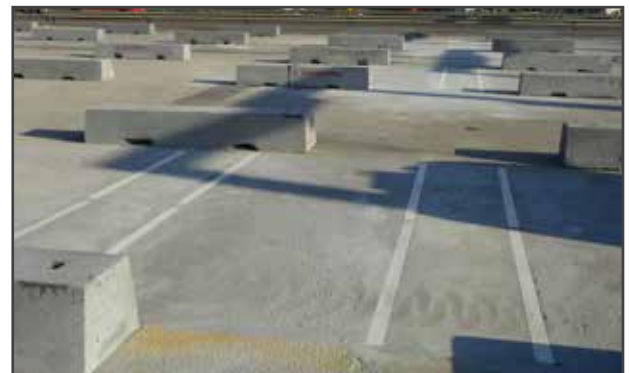
Weigh-In-Motion Strip Sensors were installed in four rows per lane for the port gate application.
