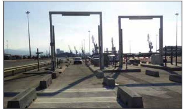
In-ground installation of port dynamic weighbridges in Thessaloniki, Greece
